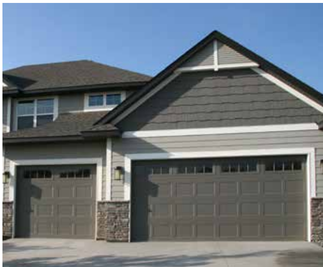
AR-II in earhttone with stockbridge windows
